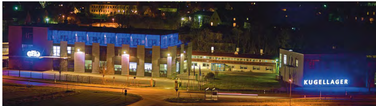
Headquarter and production site at Rimpar
